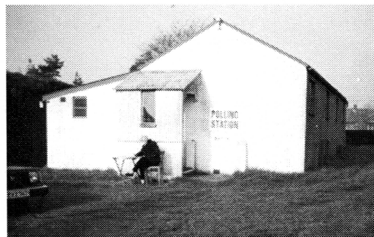
The Old Village Hall on Polling Day 1992 (A few weeks before it was pulled down)
